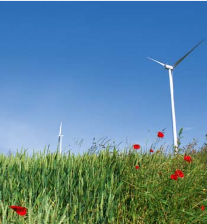
Raucourt (France) 12 MW
